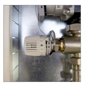
The thermostatic head adjusts the temperature of water through the flow manifolds. The temperature can be set by turning the head to the desired figure.
